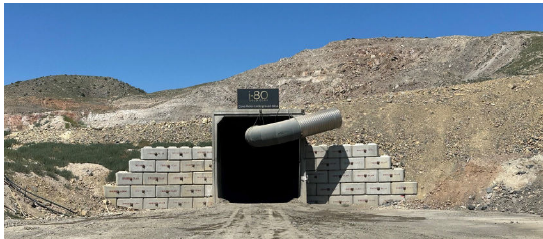
Figure 1 – Portal and Decline at Cove
