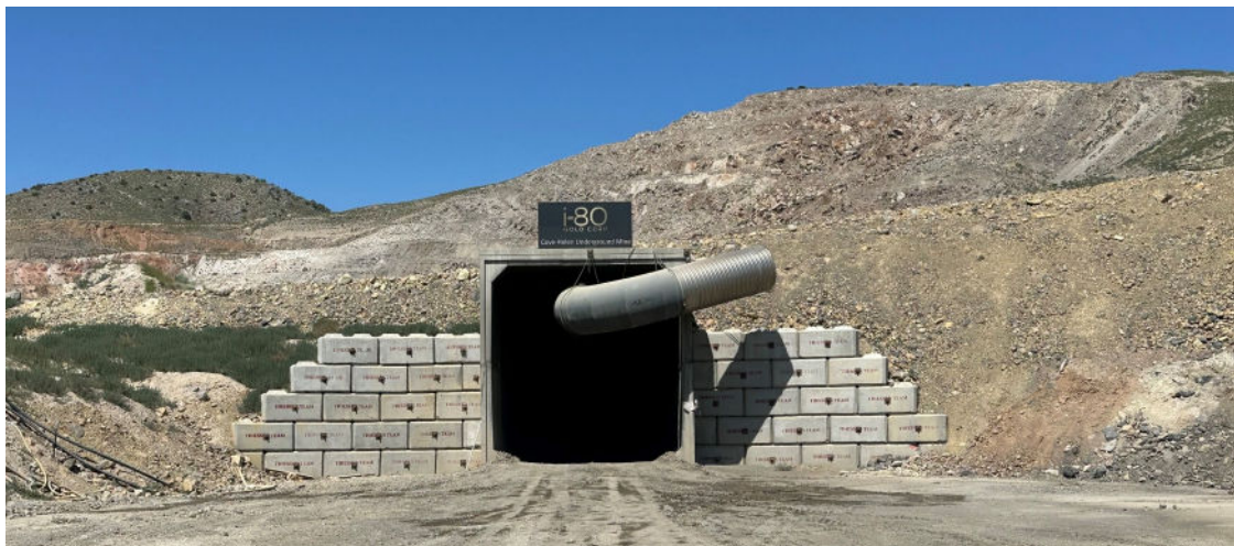
Figure 4 – Portal and Decline at Cove
