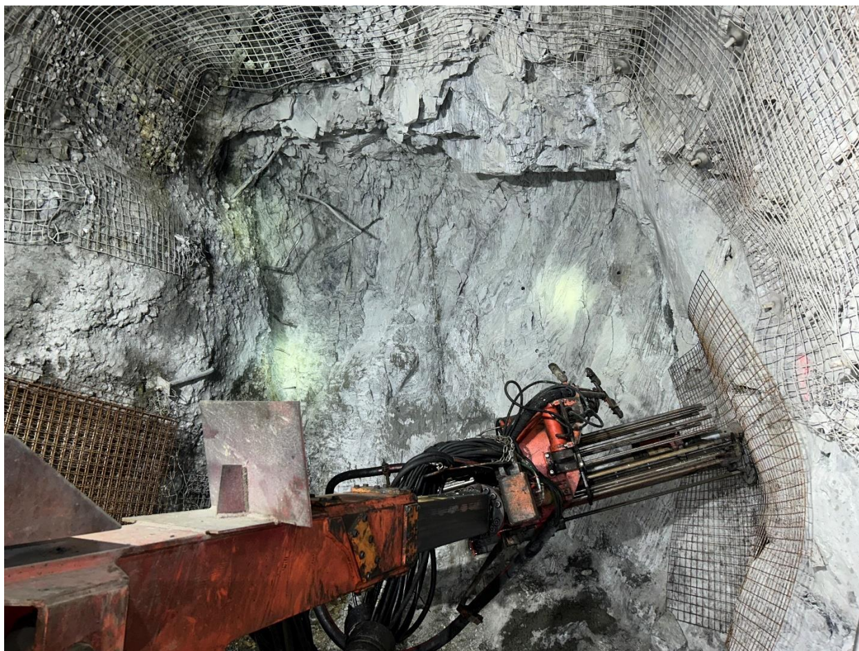
Photo 16-1: Primary Ground Support Installation
