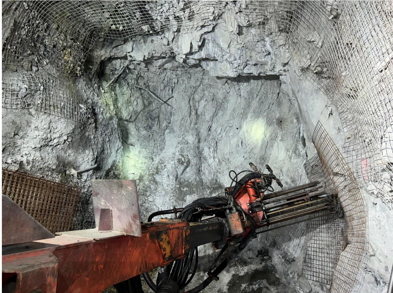
Figure 13-17 Primary Ground Support Installation
