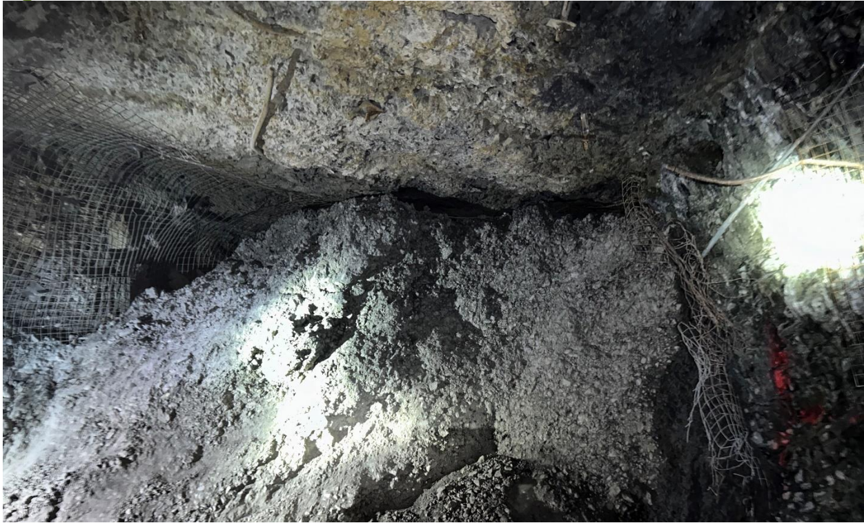
Figure 13-18 Cemented Rock Fill in Adjacent Cut
